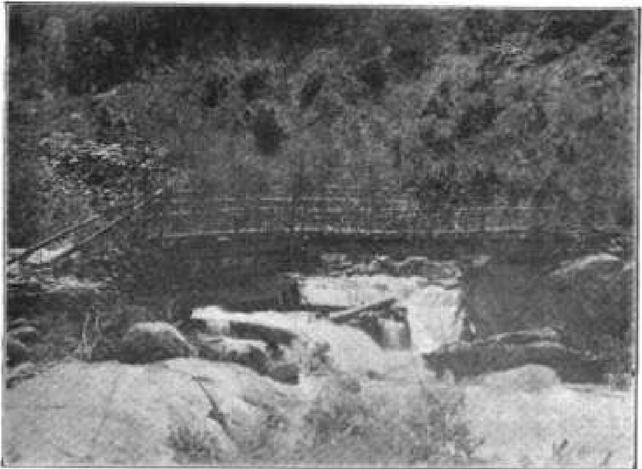
BRIDGE BETWEEN ELARAT AND ASHRETH.
