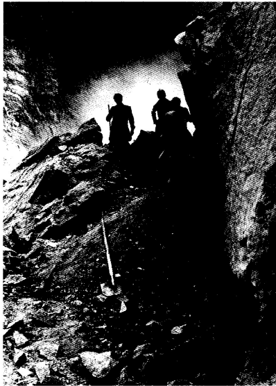
Fig. 43. The recent construction of the Aliabad irrigation channel which links the Hassanabad glacier with the fertile oasis of Central Hunza. The same rock-blowing and retaining wall construction techniques are used for building road tracks.
