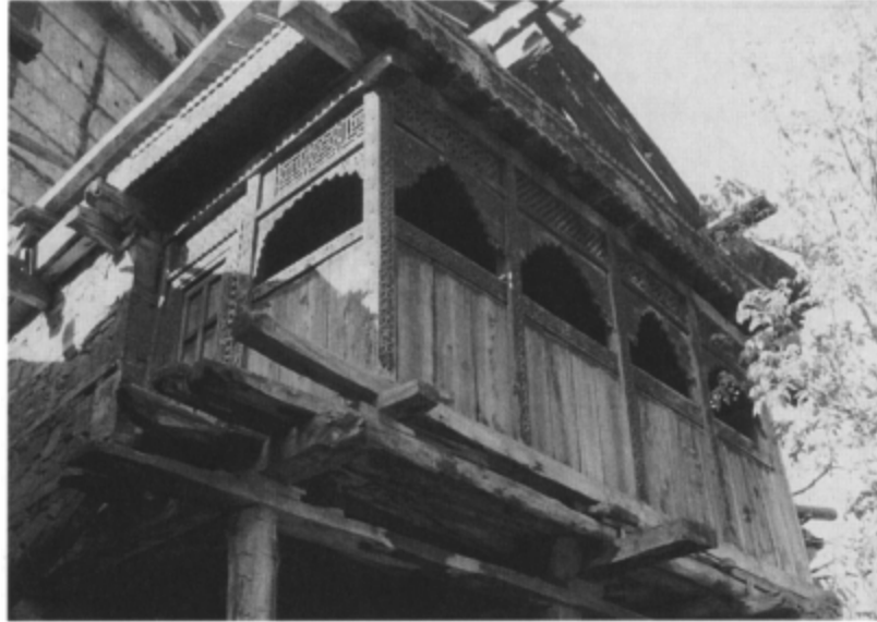
Fig. 4: House of Azimullah in Harban-kot. Veranda showing influences of Mughal architecture (multi-cusped arches and jali-screens)
